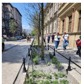
Rain gardens on Krupnicza Street in Krakow (photo: ZZM in Krakow)
