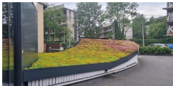
Green roof of extensive type on the entrance to the underground garage in Krakow (photo: Małgorzata Siudak)
